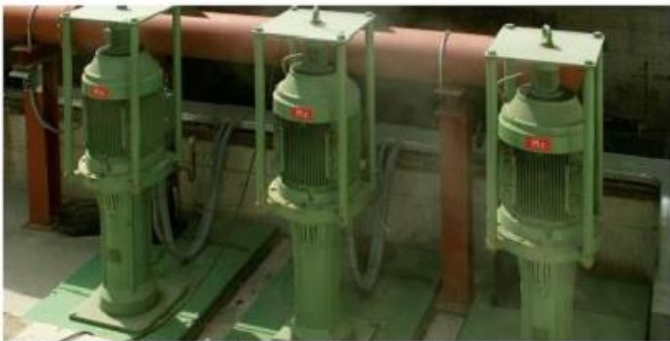
Vertical PEMO pumps for transfer of slurries
