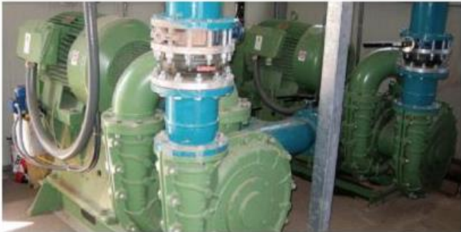
Horizontal double stage PEMO pumps for filter press
