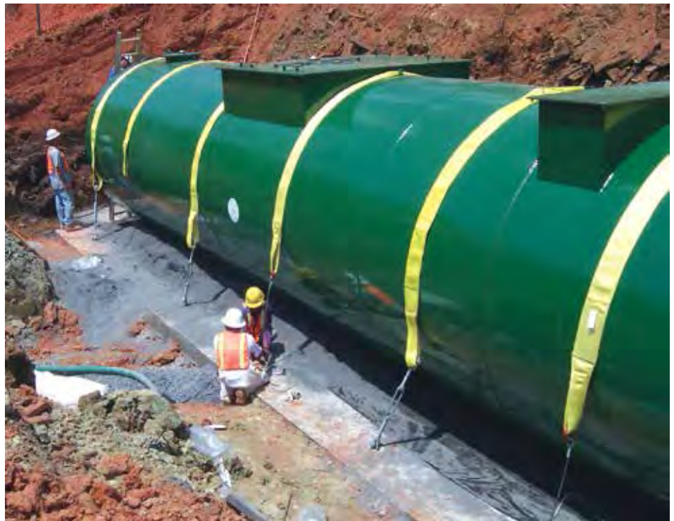
Polyester Hold-Down Straps Installation Detail
